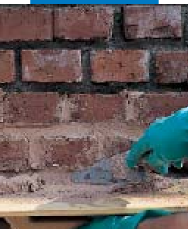
Pointing of brickwork with Mape-Antique CC
