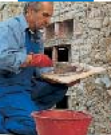
Trowelling on Mape-Antique CC mortar
