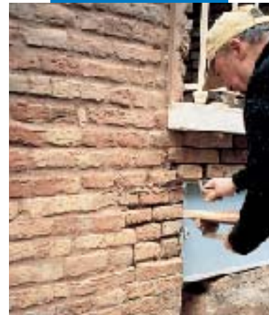
Detail of façade, Bagnacavallo, Italy
