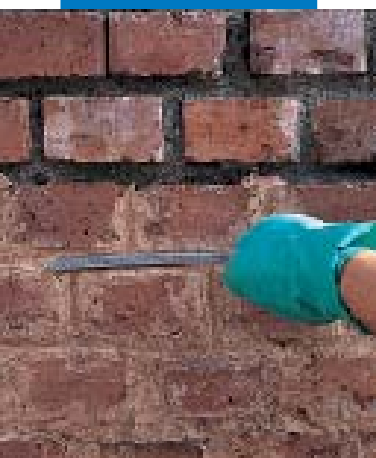
Finishing joints in a brick wall with Mape-Antique CC
