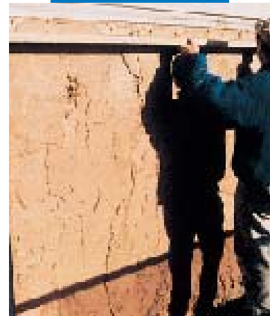
Restoring a façade with Mape-Antique CC
