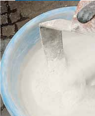
Preparation the Mape-Antique MC mix
