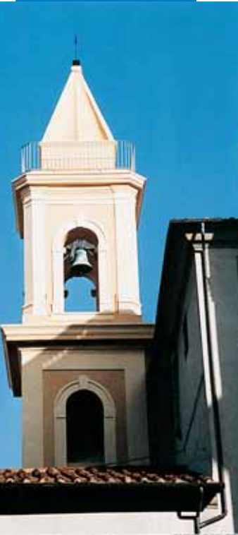
Bell tower restored with Mape-Antique MC
