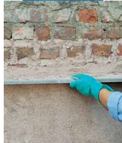
Levelling render made with Mape-Antique MC
