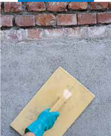
Float finishing render made with Mape-Antique MC
