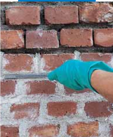
Pointing of brickwork
