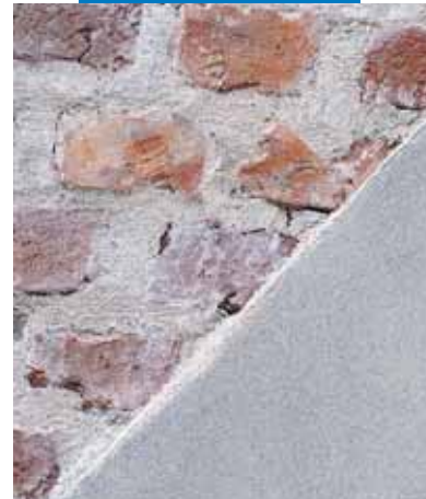
Detail: Mape-Antique MC used for filling joints and rendering
