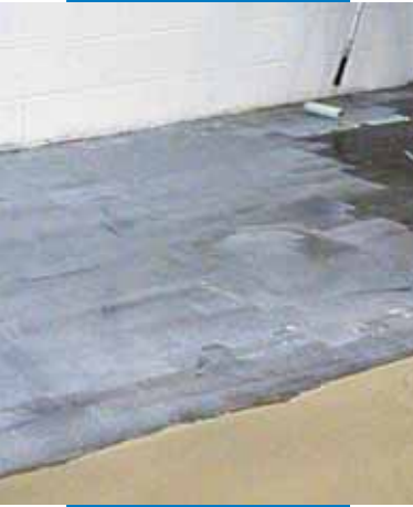
Application of Mapeprim SP
