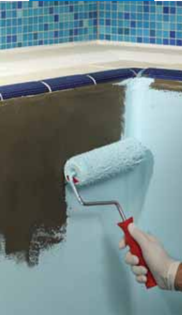
Application of Elastocolor Waterproof with a roller
