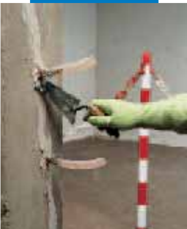
Fixing injection tubes with Adesilex PG1
