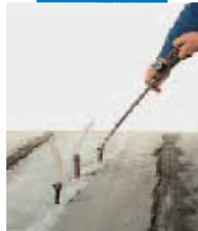
Restoring horizontal structure by injection with Epojet
