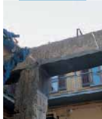
Repairing beam with injection of Epojet
