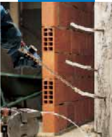
Injecting Epojet to a fissured pillar
