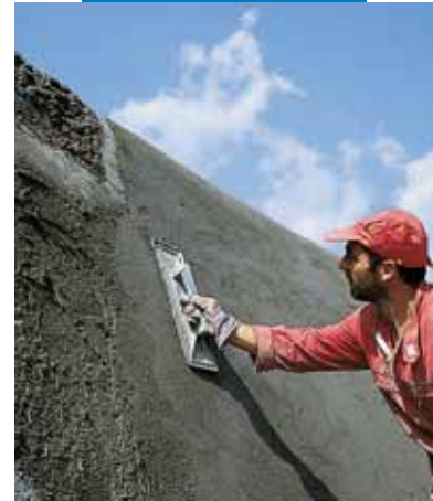
Finishing of Mapegrout T40
