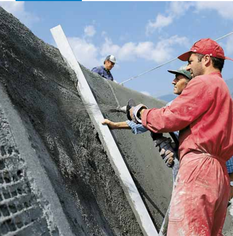
Spray application of Mapegrout T40
