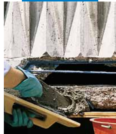
Repairing a balcony with Mapegrout T40
