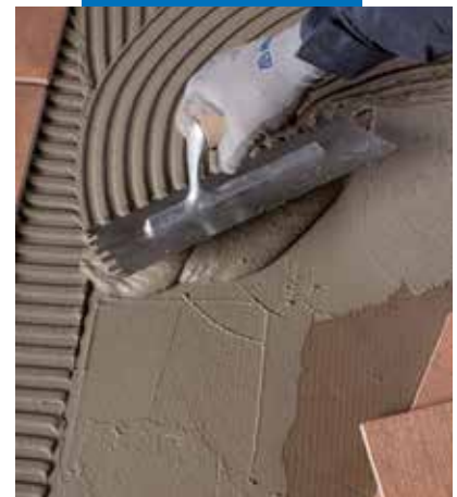
Bonding tiles with Elastorapid
