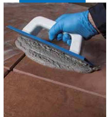
Grouting tiles with Ultracolor Plus
