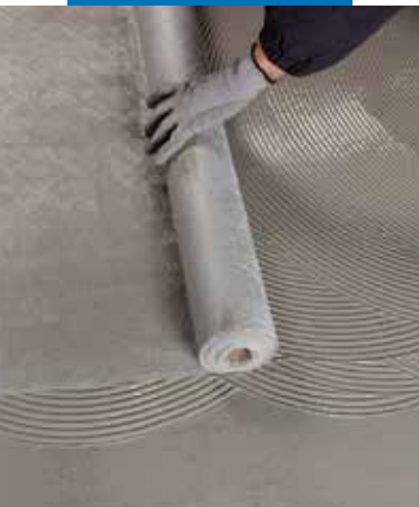
Placing Mapenet Sel on the first layer of Mapelast ic Turbo while wet
