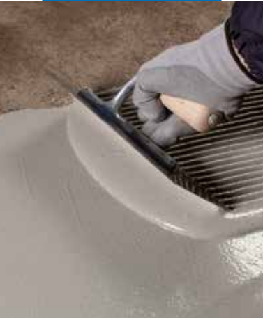
Application of the first layer of Mapelast ic Turbo
