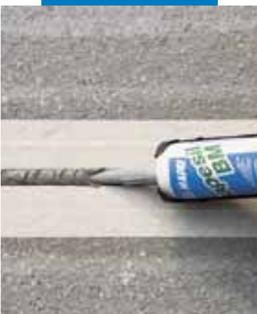
Joint filling with Mapesil BM
