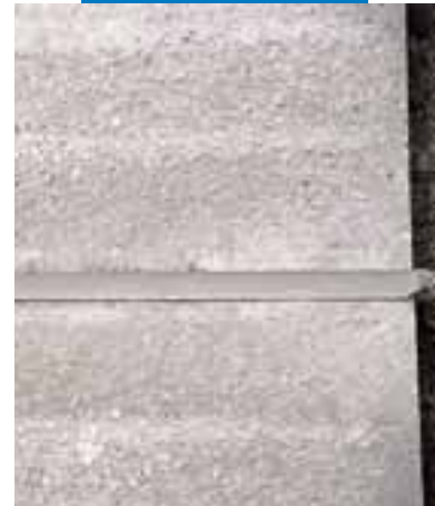
Final sketch of the joint after removing the protective tape
