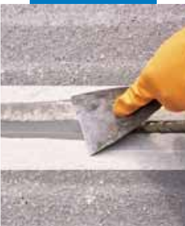
Joint smoothing by removing the excess sealant
