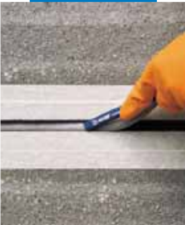
Protection of the joint edges with a protective tape and positioning Mapefoam into the joint
