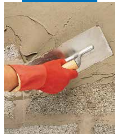
Application of Planiseal 88 by trowel
