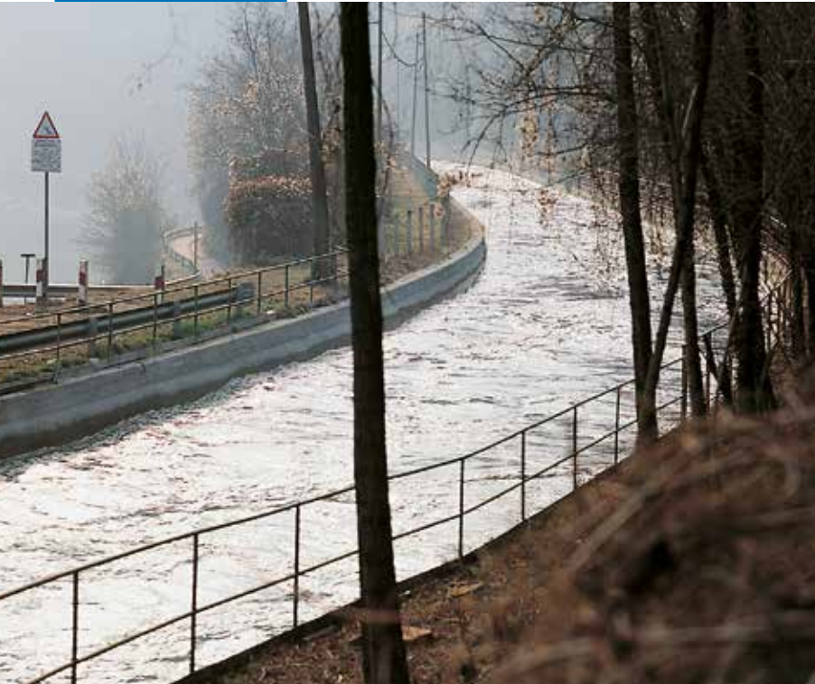
Bertini hydroelectric canal - Como - Italy. Surfaces treated with Planiseal 88
