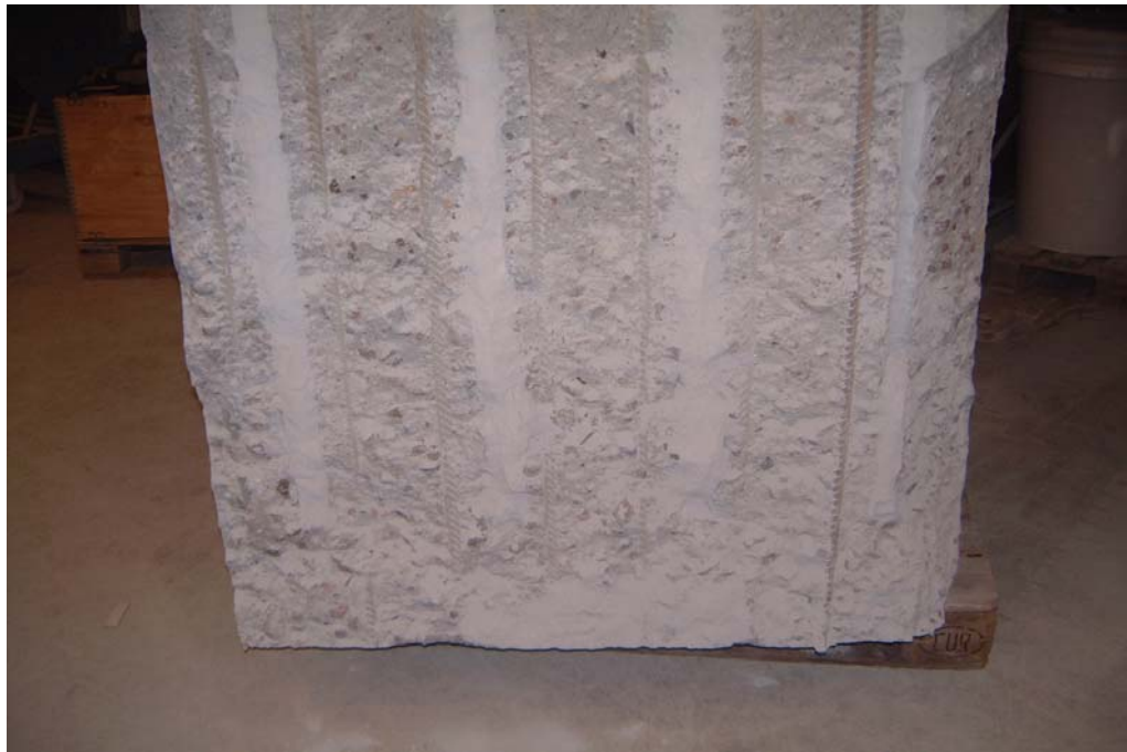
Figure 4:5 Section at second reinforcement row in relation to placing of the tremie pipe.
