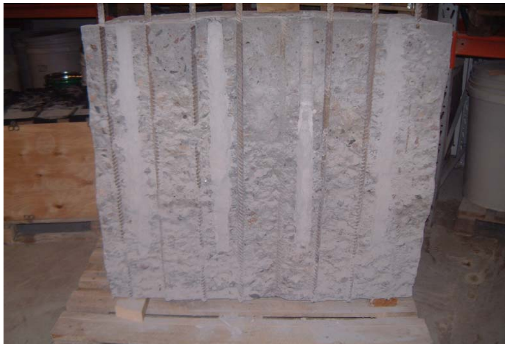
Figure 4:4 Section at first reinforcement row in relation to placing of the tremie pipe.
