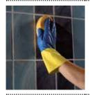
Remove any excess liquid from the surface with a hard, cellulose sponge (such as a MAPEI sponge). Replace the sponge when it is too impregnated with resin. It is important that there are no traces of grout on the surface of the tiling after the cleaning operation. Once hardened it is very difficult to remove, whichh is why the sponge must be rinsed frequently.
