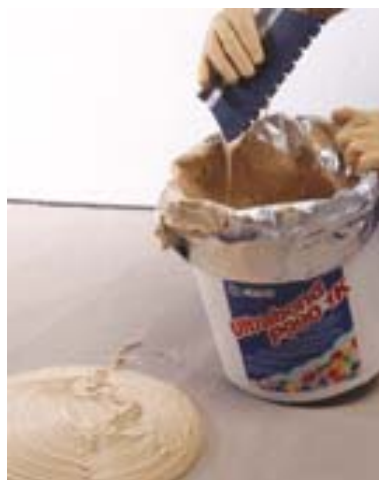
Cleaning off the adhesive from the bucket with a trowel
