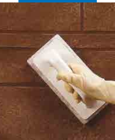
Ultracolor Plus paigaldamine seinale kummist silutiga
