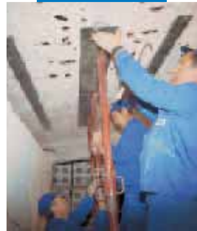
Placing metal sheet for structural reinforcement
