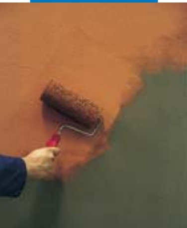
Example of an application of Elastocolor Rasante with a porous sponge roller
