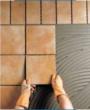
External installation of klinker tiles
