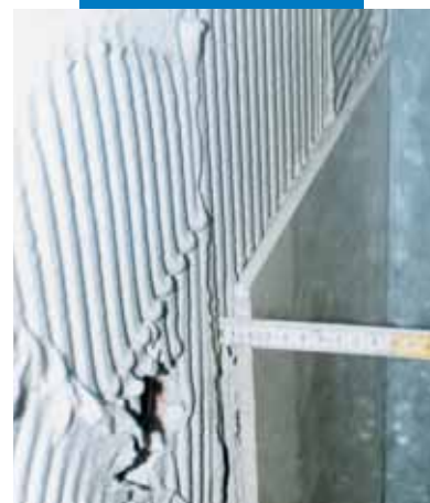
Thickly applied porcelain tiles on a wall
