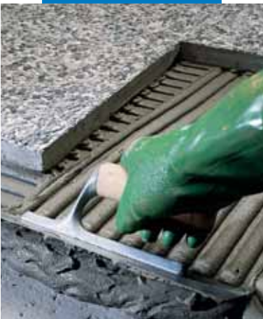
External installation of relief terrazzo "graniglie" tiles
