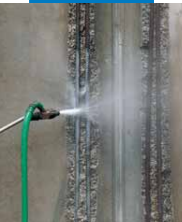
Cleaning reinforcing rods
