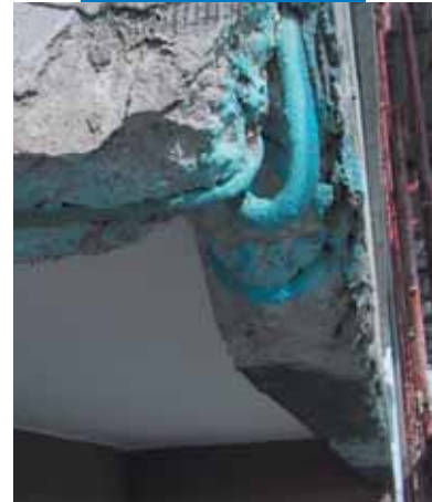
Reinforcing rods of the front side of a balcony treated with Mapefer 1K
