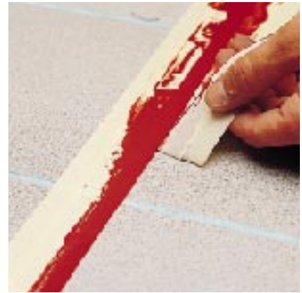
Removing the masking tape from the joint
