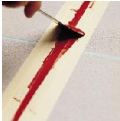
Smoothing the joint
