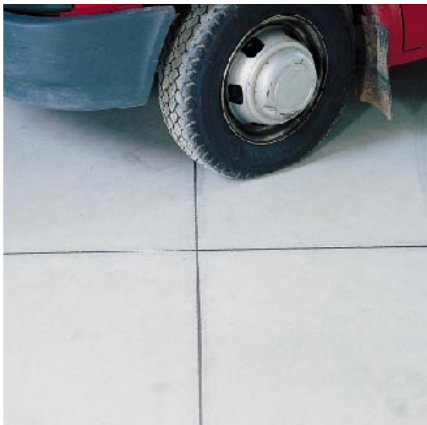
Movement joints of an industrial concrete floor sealed with MAPEFLEX PU21
