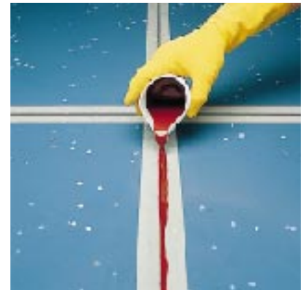
Filling a joint between rubber floor tiles
