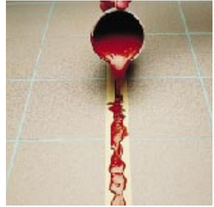
Filling the joint with MAPEFLEX PU21
