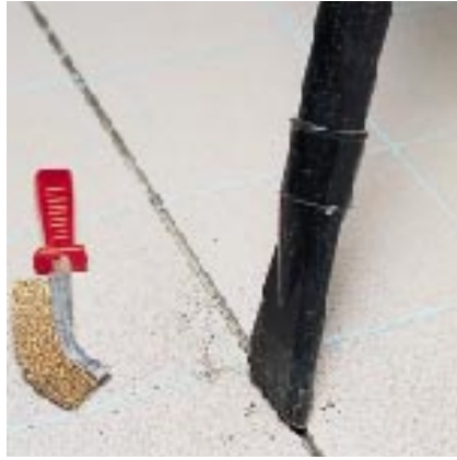
Cleaning out the joint with a dust extractor
