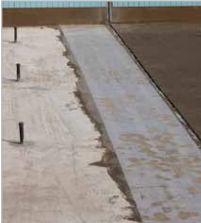
Fig. 3.10 - Waterproofing treatment with MAPELASTIC SMART and MAPETEX SEL
