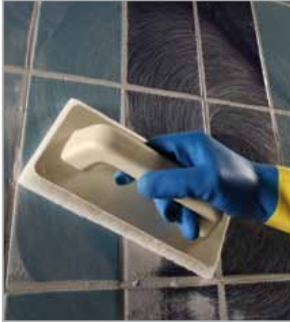
Fig. 5.7 - Cleaning the surface of the lining with a Scotch-Brite® pad
