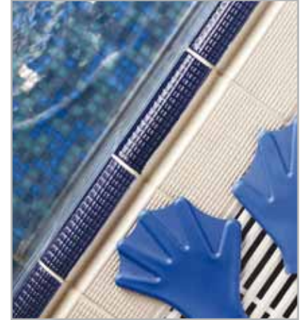
Fig. 5.5 - Grouting the lining with ULTRACOLOR PLUS
