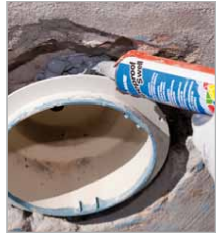
Fig. 4.2 - Forming a seal with MAPEPROOF SWELL
