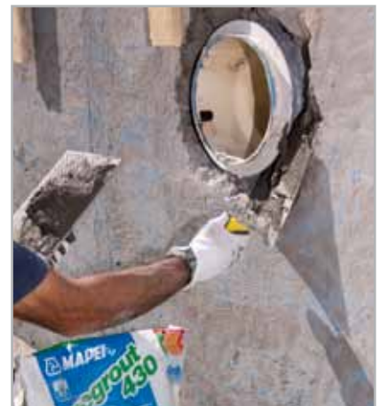
Fig. 4.3 - Reintegrating a substrate with MAPEGROUT 430
