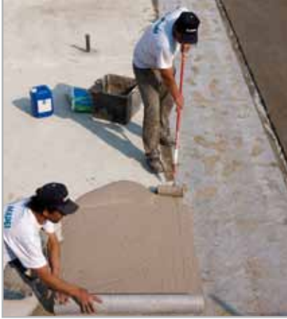
Fig. 3.9 - Waterproofing treatment with MAPELASTIC SMART and MAPETEX SEL
