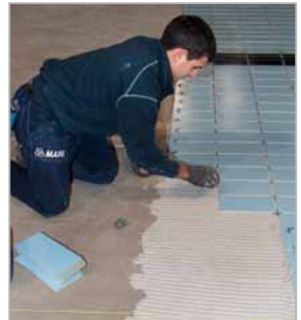
Fig. 5.3 - Installing the lining on the bottom of a swimming pool
