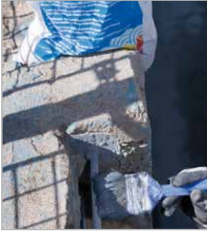
Fig. 4.1 - Applying a coat of MAPEFER 1K on reinforcing bars
