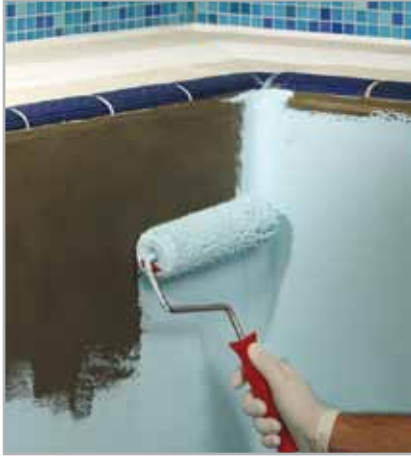
Fig. 6.2 - Applying ELASTOCOLOR WATERPROOF with a roller
