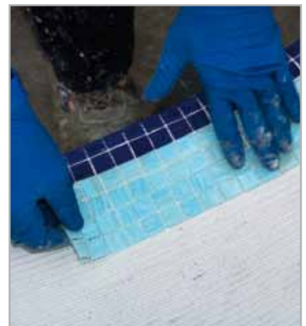
Fig. 5.4 - Installing a mosaic lining
