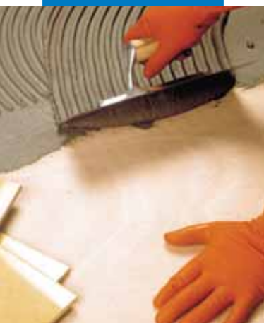
Laying porcelain tiles on a marine plywood substrate with Elastorapid
