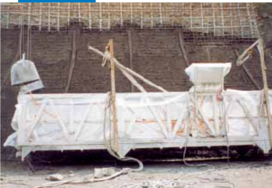
A detail of a concrete surface during repair
