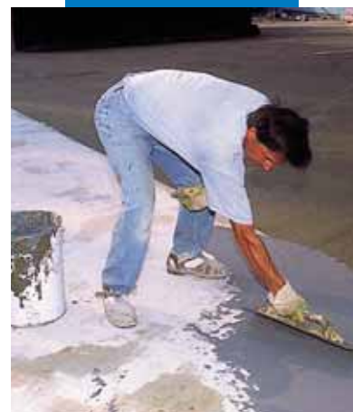
Waterproofing a swimming pool with Mapelastic
