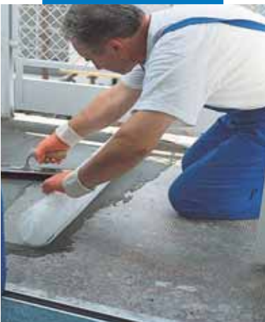
Waterproofing a balcony with Mapelastic incorporating Mapenet 150 reinforcement
