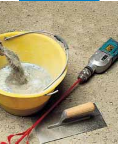
Mixing Mapelastic with a mechanical mixer
