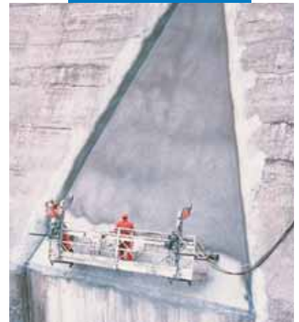
Example of Mapelastic applied on a dam by spraying
