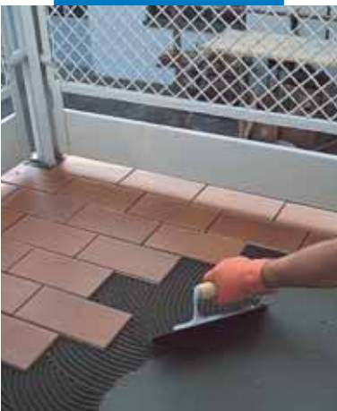
Fixing tiles with Granirapid onto a balcony waterproofed with Mapelastic
